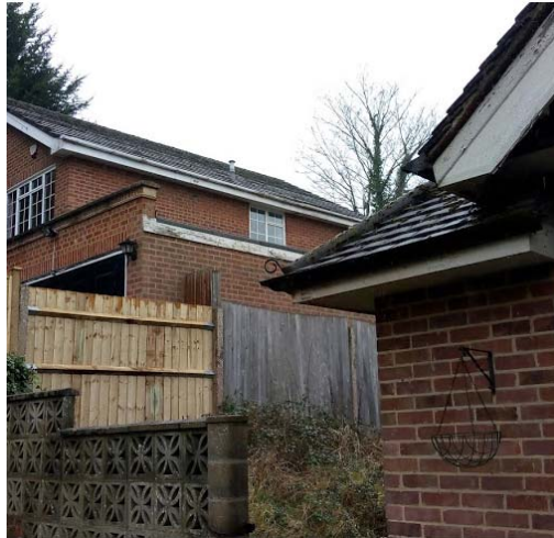
(Photo A – Site Photo of Flank Elevation of 61A)
