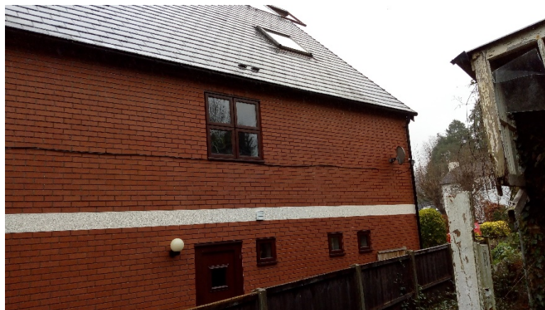
(Photo B – Site Photo of Flank Wall of no.65)
